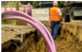
12 to 14 bar: Cable blowing and drilling
