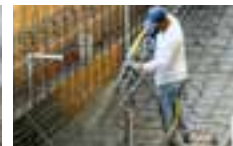
7 to 12 bar: Shotcrete applications
